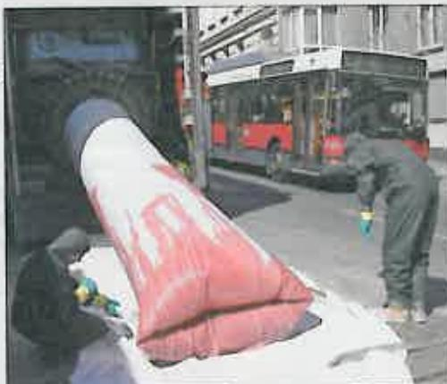
The new r.tec® W2 Inliner, a special Rabmer development for drinking water pipes, is ready for being pulled into the old pipe (Vienna, 19th district, Barawitzkagasse)
